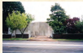
Latingata Morrum Centre (gym) being built
